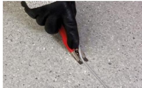
1<sup>st</sup> pass with a Mozart knife with a spacer
