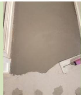
Any repairs to a timber subfloor as a result of a flood or water damage will need the joists to be moisture tested; including new joists. Moisture in timber takes considerable time to dry. If the joists are not sufficiently dry, shrinkage will cause movement of the structural sheet. Screw/nail holes may protrude and show through the resilient floor covering.
