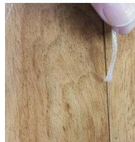
Before applying the chemical weld, the seams should be first masked with tape to slow down the application process. This will allow time for the chemical to run into the seam and bond the sides together. The tape should then be removed before the chemical dries.
