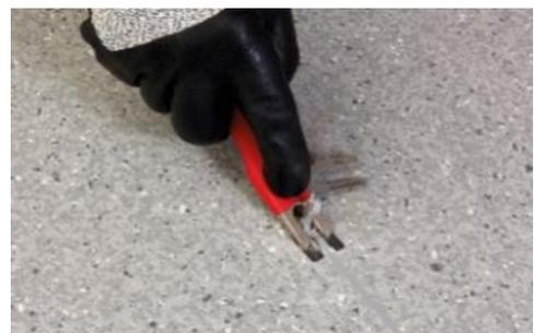
2<sup>nd</sup> pass with a Mozart knife without the spacer
