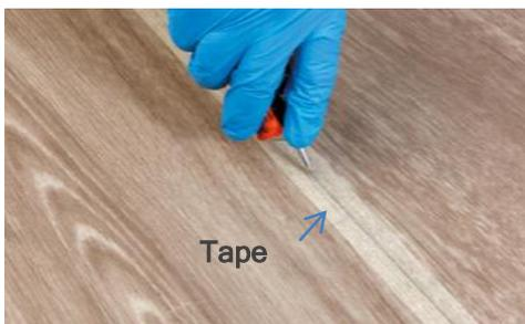
Photo 1: Applying a clear liquid chemical into the seam that side bonds the seam together (polyflor).
