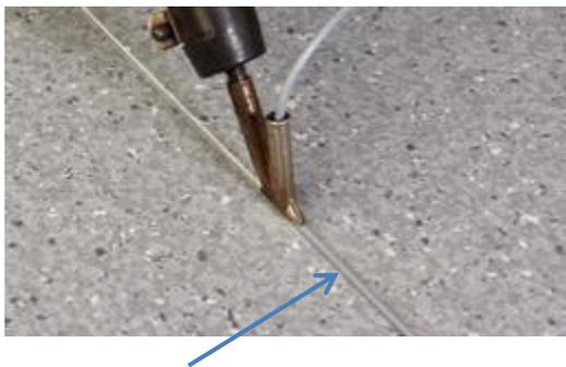
A slight **wash** of melted weld rod rising at the edge of the weld
