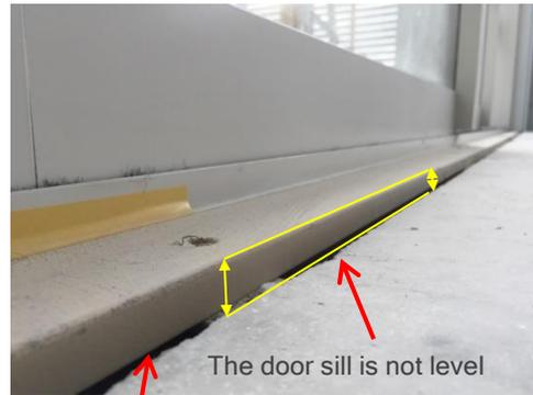
A gap between the concrete and door sill will not allow the vinyl floor covering to finish neatly against it.
