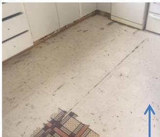
**Photo 1** Vinyl wear layer separated from its backing
