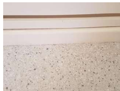
Photo 4 - After vinyl is fitted any excess silicone that squeezes up is removed.
