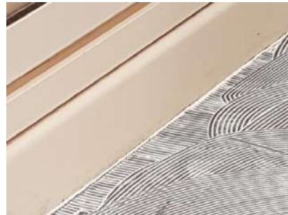
Photo 3 Silicone to the shower/floor junction.
